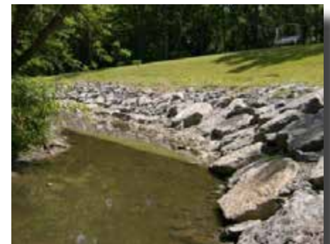
Stream bank after stabilization
