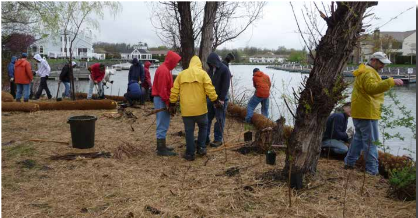
Atwater Meadows shoreline stabilization project. Project completed with the Canandaigua Tennis team installing the plantings and coir rolls to stabilize shoreline.
