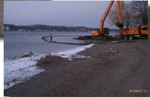
Deep Run dredging in progress (below).
