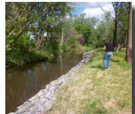
Parrish Street Stabilization
