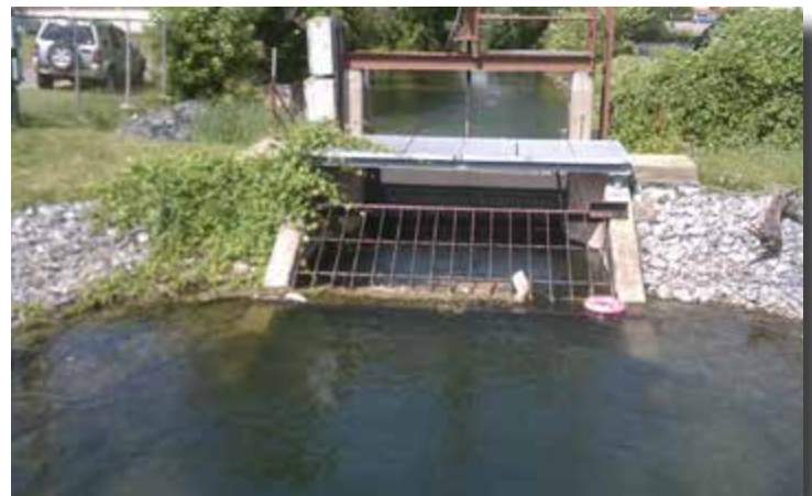
The feeder canal allowing the minimum flow out.
