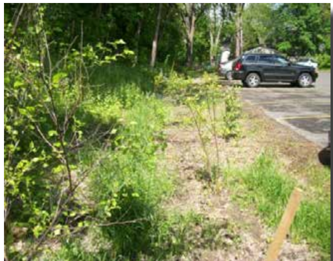
YMCA bio-retention facility
