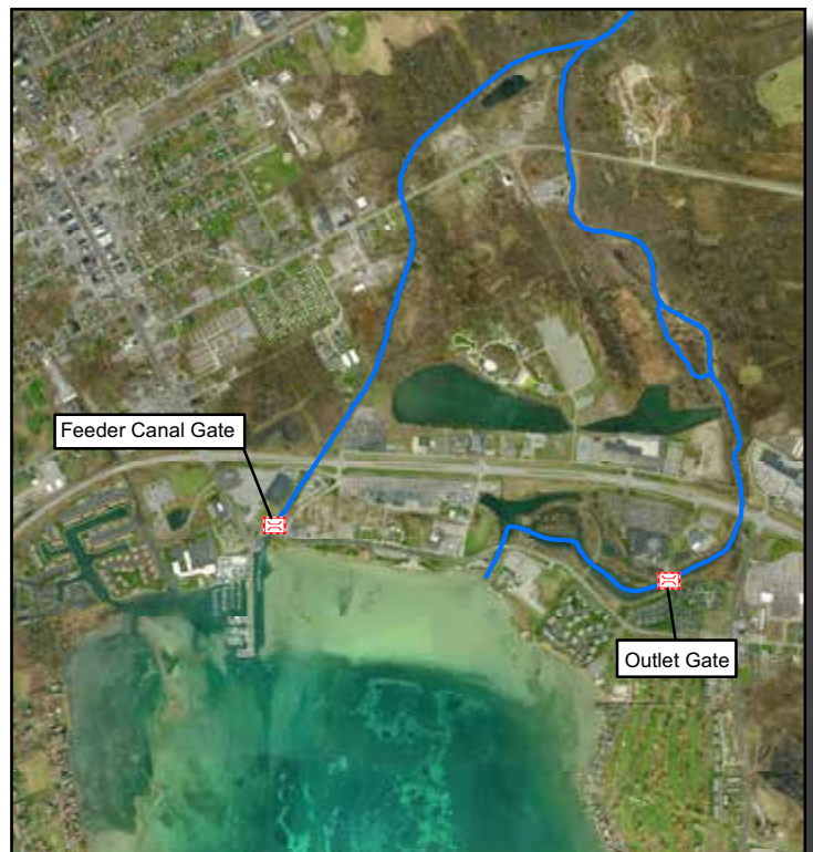
Location of the Feeder Canal and the Main Outlet Gates
