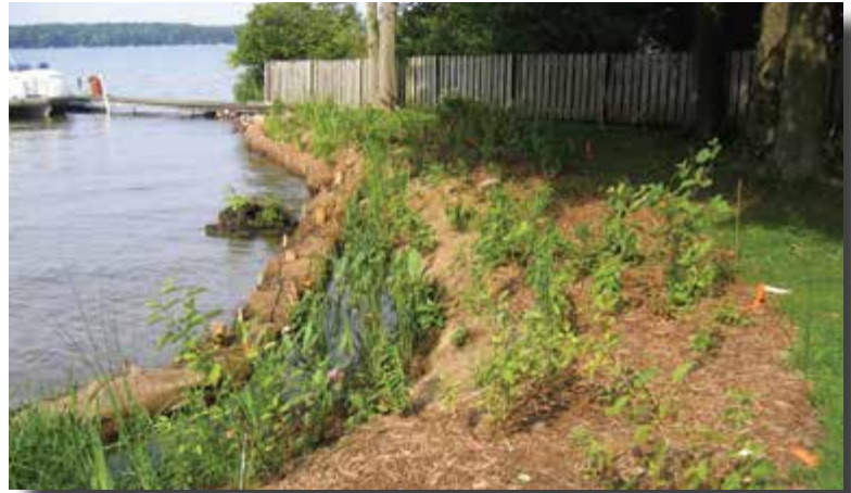
Example of a vegetated shoreline buffer. Photo from Natural Shorelines for Inland Lakes, a publication produced by Michigan Sea Grant and the Michigan Department of Environmental Quality.
