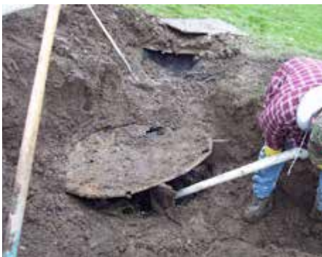
Digging up a failed onsite wastewater system.
