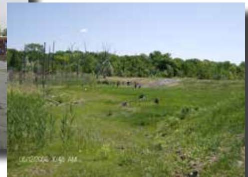
Canandaigua School District stormwater wetland
