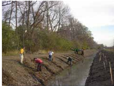
Outhouse Town Park stream stabilization project utilizing willow wattles.
