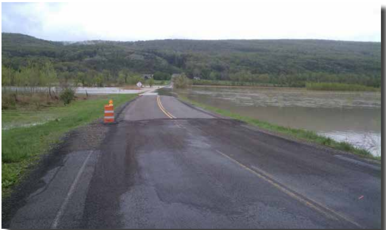
Naples Creek flooding Parrish Flats Road during May 2014 storms
