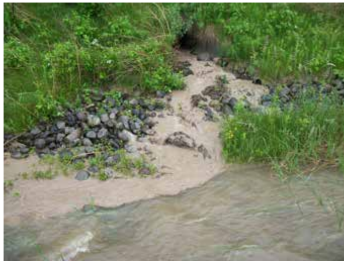
Muddy runoff coming from a development site.
