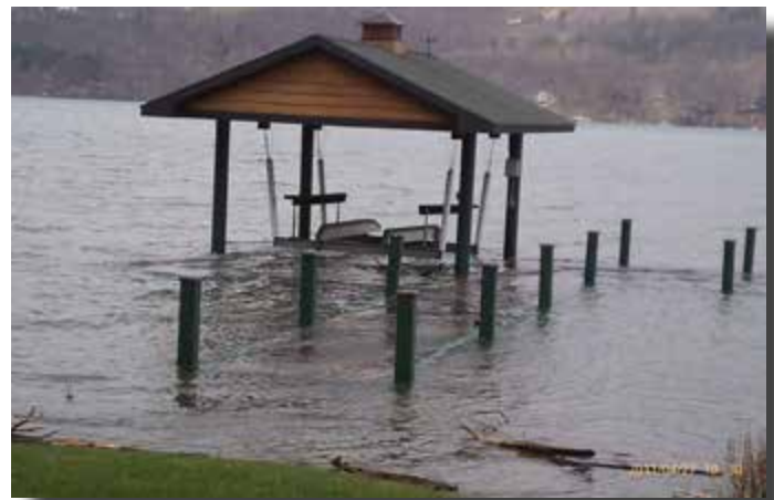
Flooding along the lakeshore
