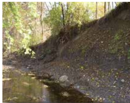
Stream bank before stabilization
