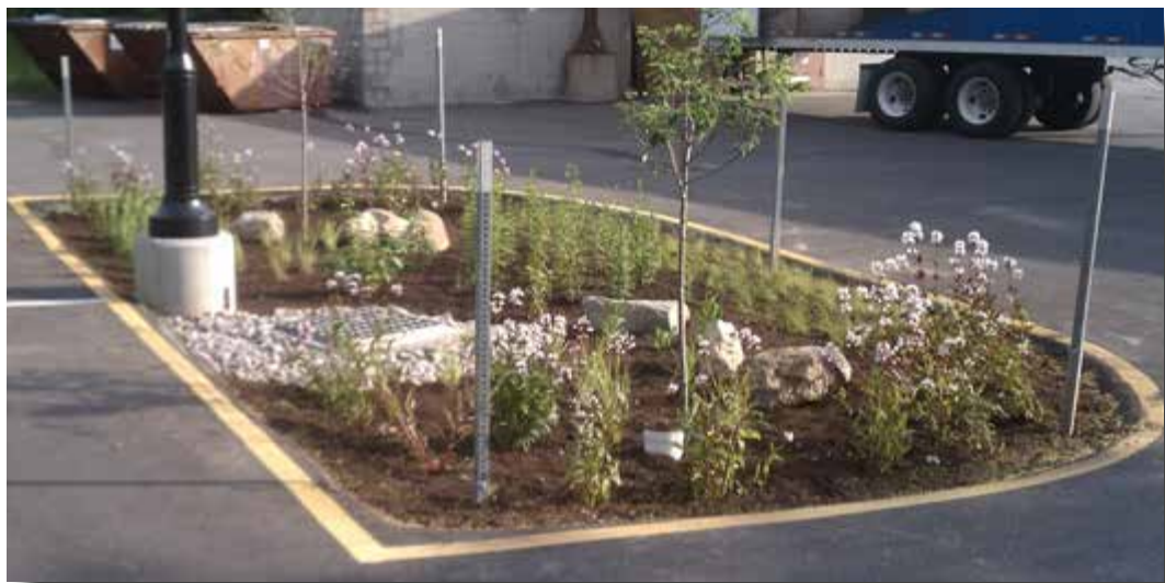
Antis Street Parking Lot- bio-retention areas
