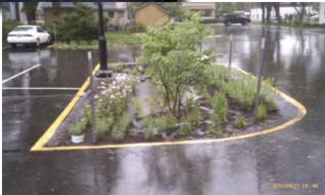
Antis Street - before (left) and with a bio-retention project in action (above)
