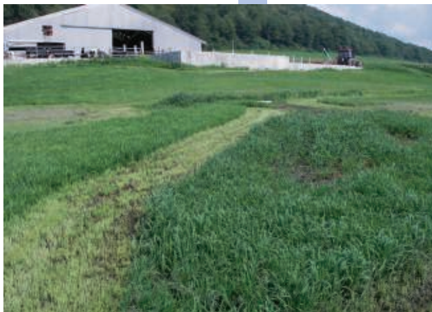
A buffer is designed and installed to capture and filter barnyard runoff.
